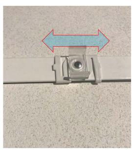
Once Clip is installed slide trough the T-Grid until it is located in the right position.
